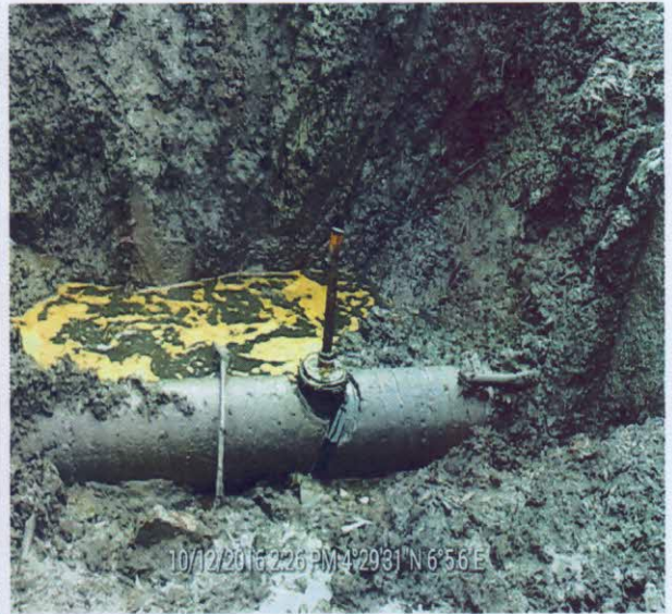
Fig 4: Pegging of spill point
