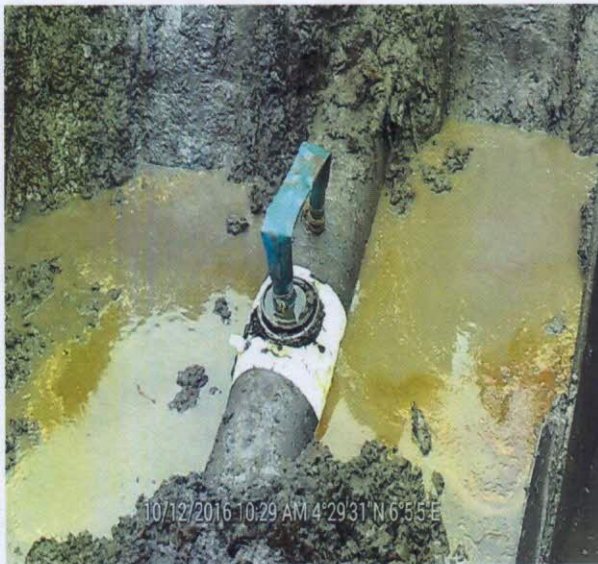
FIG 3: Spill point after excavation
